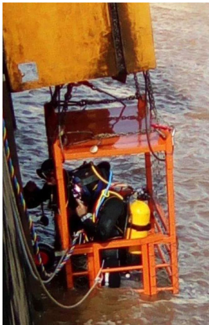
Divers in Songloulou spend several hours under water to seal cracks
