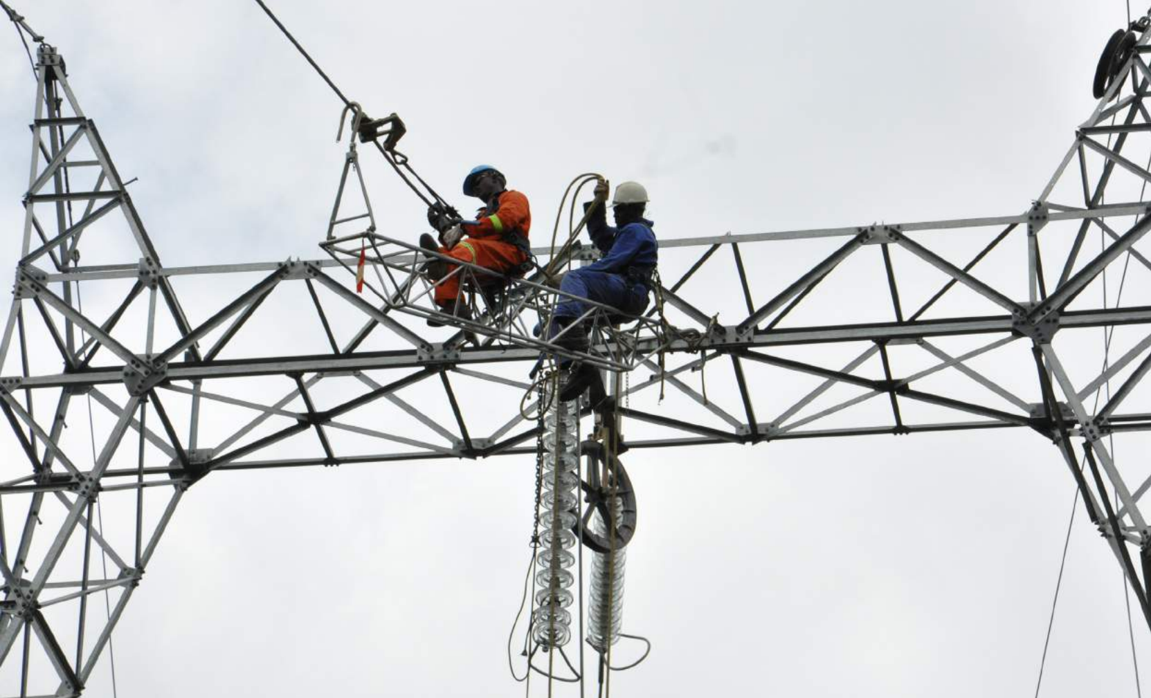
The line Mangombé-Oyomabang equipped with devices to scare crows
